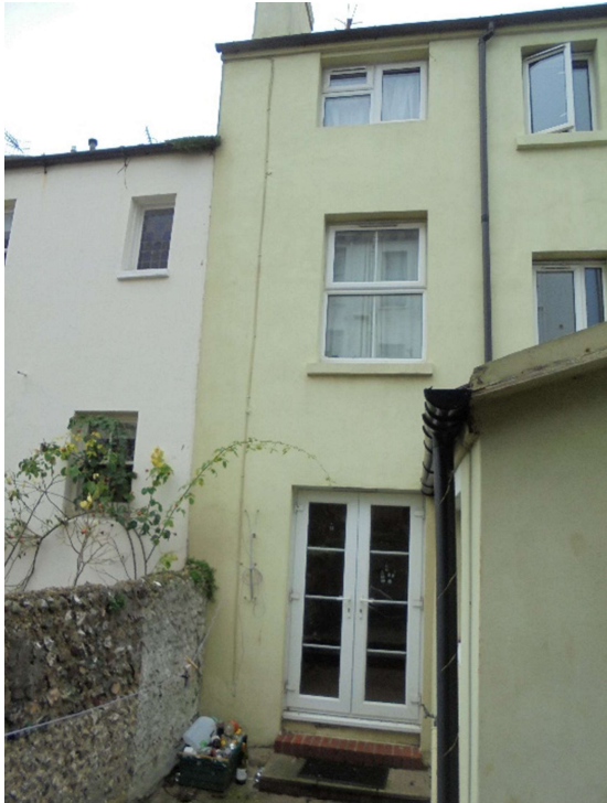
Looking to rear elevation existing extension to right
